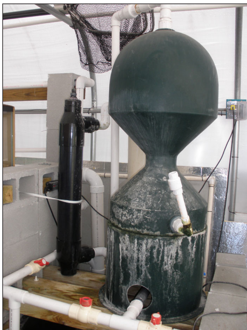
Figure 4. Life support components for a small recirculating system. Bubble-washed bead filter (which functions as both mechanical and biological filtration) and UV sterilizer unit.
