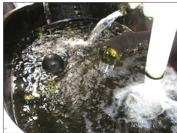
Figure 5. Sump from RAS. Depending upon design, sumps can build up significant amounts of debris, which can harbor disease-causing organisms. Sumps require periodic cleaning.
